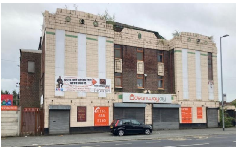
Existing building when viewed from Kenyon Lane
