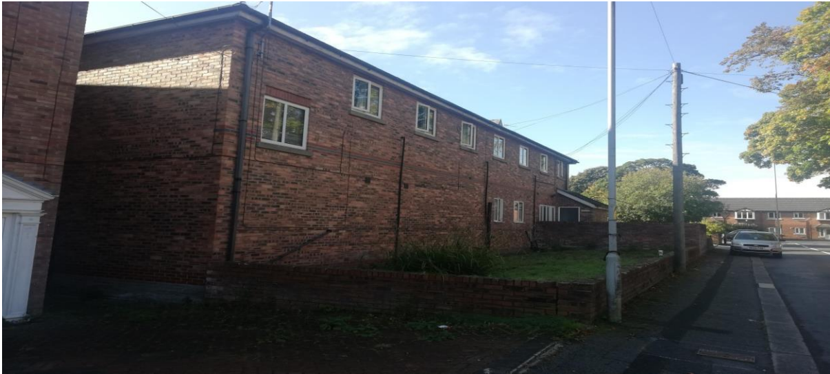
(Image 3) Building at the Junction of Middleton Road and Ardern Road south west of the site.
