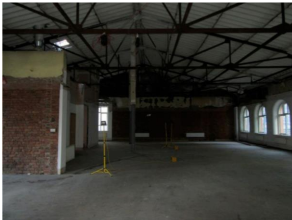
Internal view floor two
