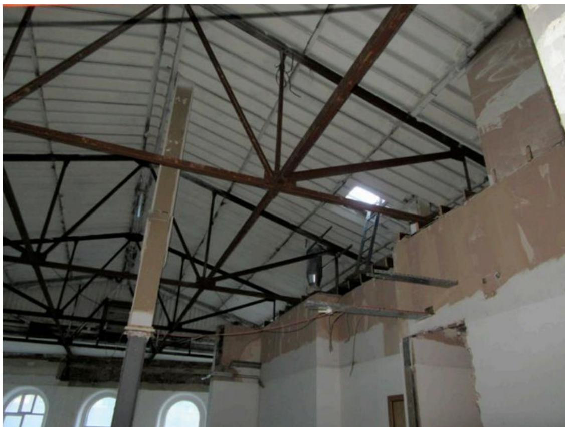
Internal view of non-original roof structure
