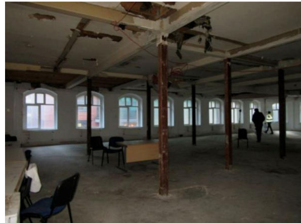
Internal view floor three
